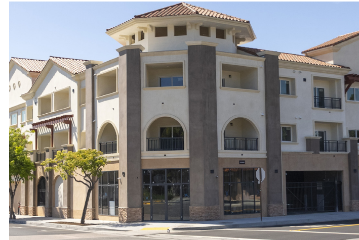
15901 Main St, La Puente. Corner of the development designed to differentiate the corner.
