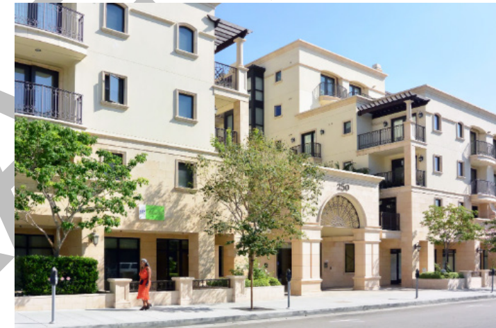
6.4: Building entry accentuated with wall articulation, massing break and portal interior courtyard
