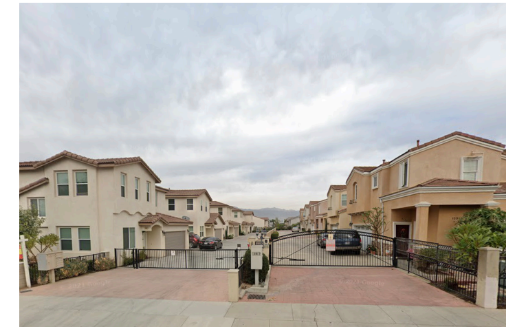
Older townhome development in La Puente
