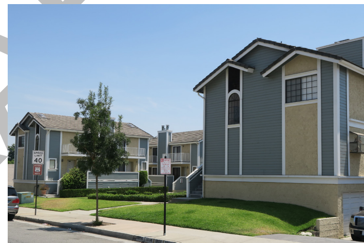
Lack of relationship between units and frontage
