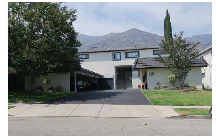
Large portion of frontage dominated by surface parking and a driveway
