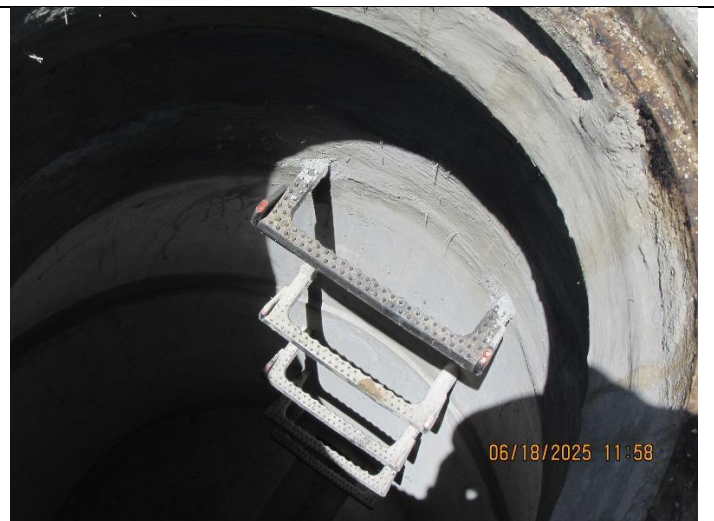
Photo 2: Composite steps with mini reflectors inside newly installed manhole.
