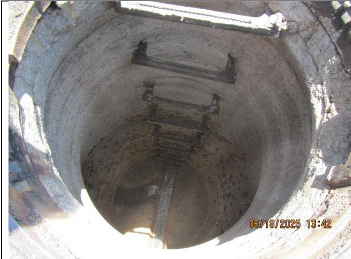
Photo 20: View inside concrete manhole with rough interior and composite steps.
