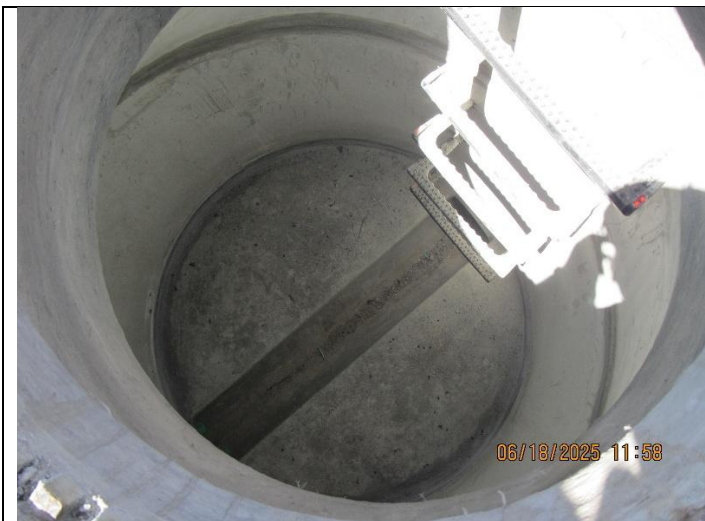
Photo 1: View inside the newly installed manhole showing minor debris in channel.
