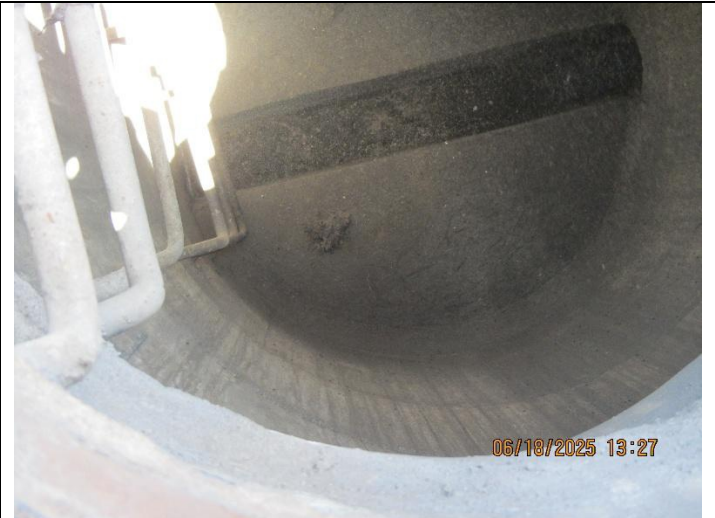
Photo 17: Cobwebs, minor debris on bench, and no flow through channel.
