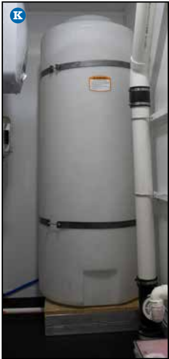
On-Board Fresh Water Tank —105 gallons
