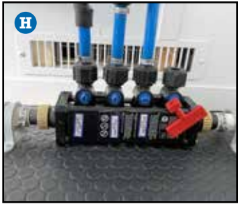
The Water Flow Control Center (main manifold) is where operator will adjust setting for City Fill or On-Board Water Supply
