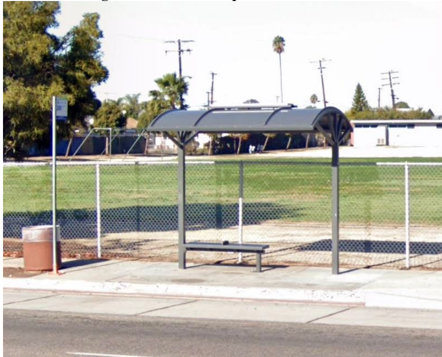
Figure A: Phase 1 Replacement Shelters
