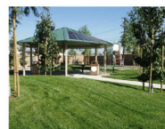
PICNIC PAVILIONS WITH ROOF SOLAR PANELS
