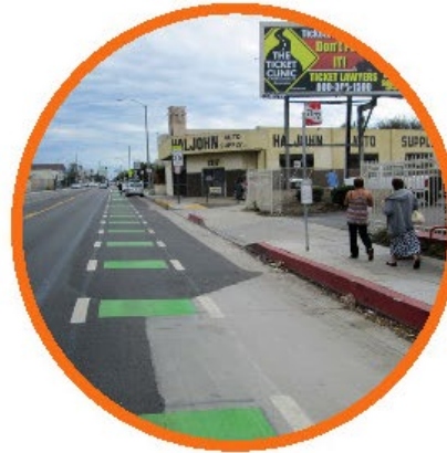
COLOR PAVEMENT TREATMENT Green Conflict Striping
