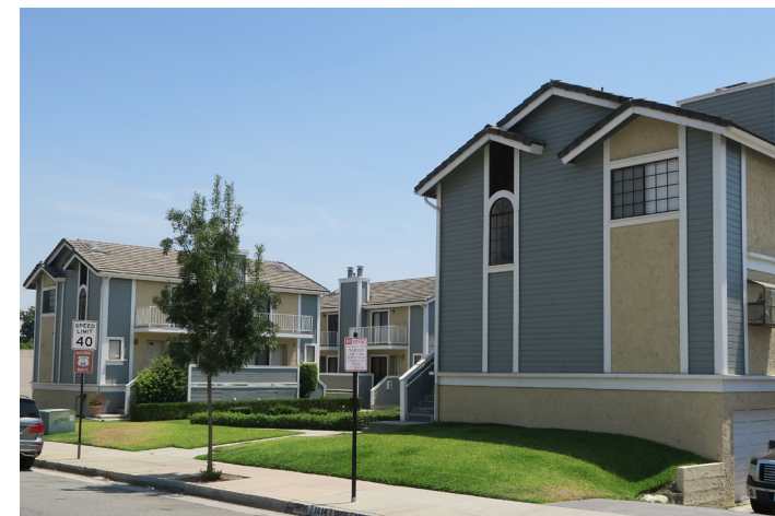
Lack of relationship between units and frontage
