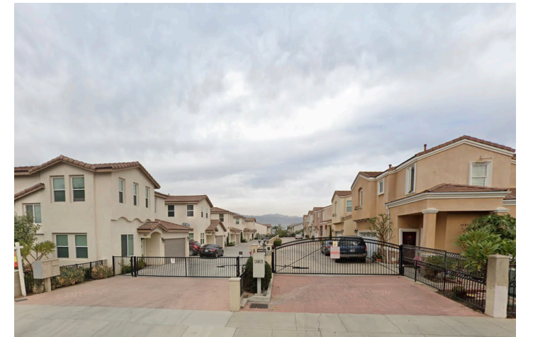
Older townhome development in La Puente
